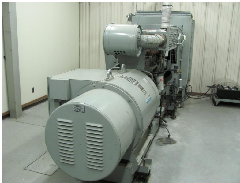
150 KW back up diesel generator powered by a Cummins engine
