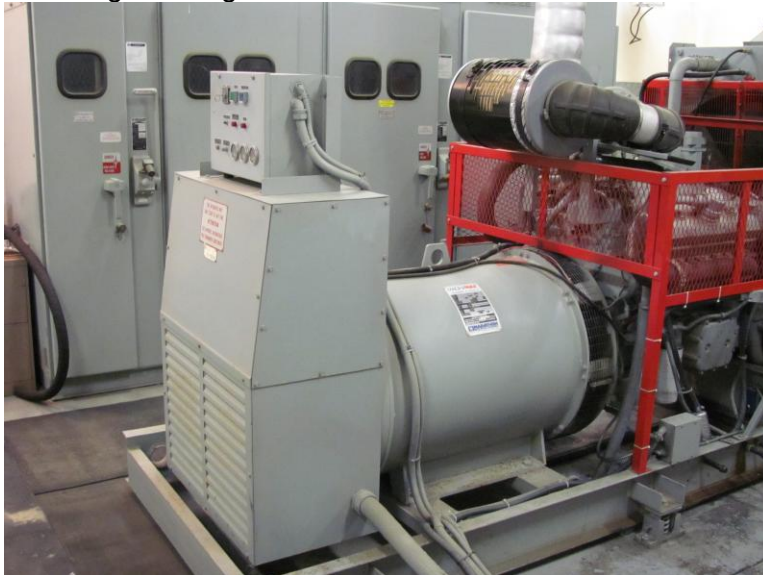
300 KW Generator with Detroit Diesel engine
