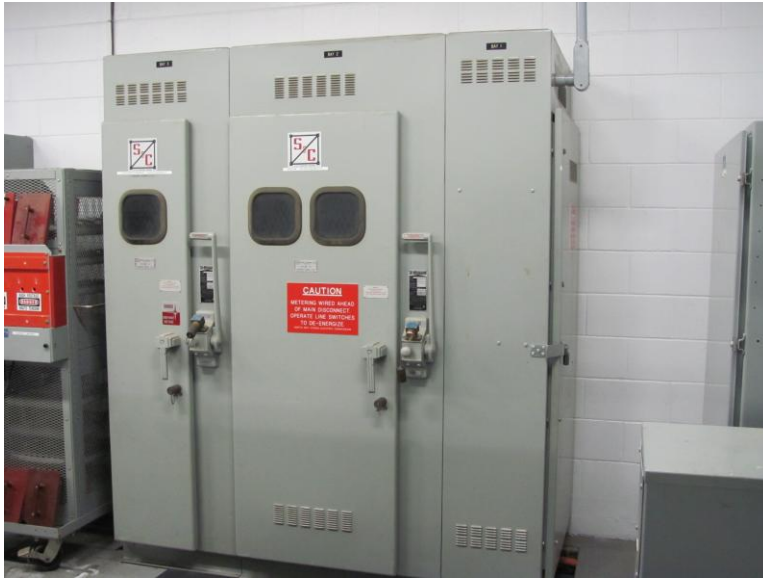
Incoming switch gear 3 cabinets Cat # 34510R5-T3
