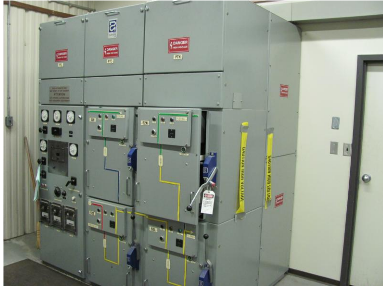
PCG Switch Gear type roll arc 400D
