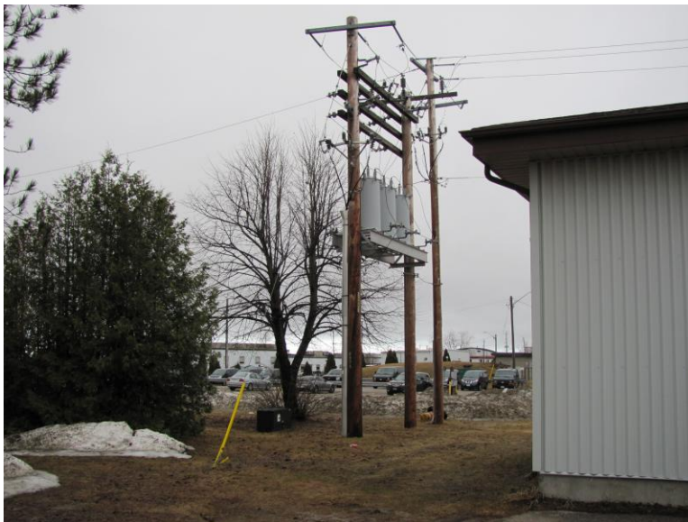
North Bay Hydro 12,880 V feed and airport's step down transformer
