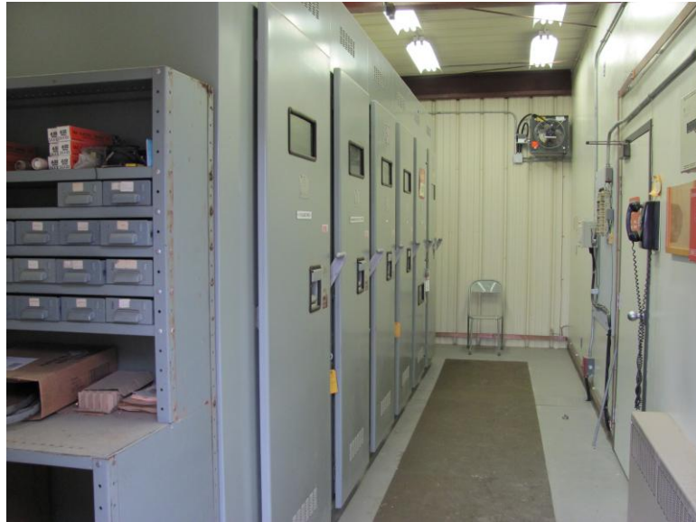
Distribution Cabinets, 1 IPU main switch, 2 Administration Building, 3 Terminal Emergency Power, 4 Maintenance Garage, 5 IPU building 6, ILS and VOR/DME
