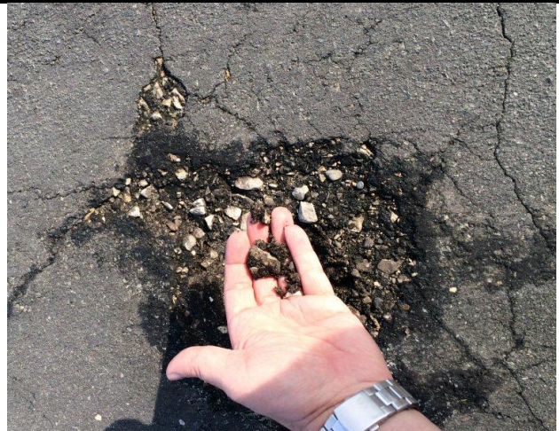
Figure 2 Soft Asphalt in Raveled Areas on Runway 06-24
