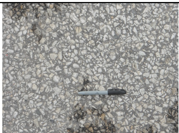
Figure 3 Surface Raveling in Location without Micro-surfacing
