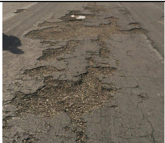
Figure 1 Surface Raveling in Location with Micro-surfacing
